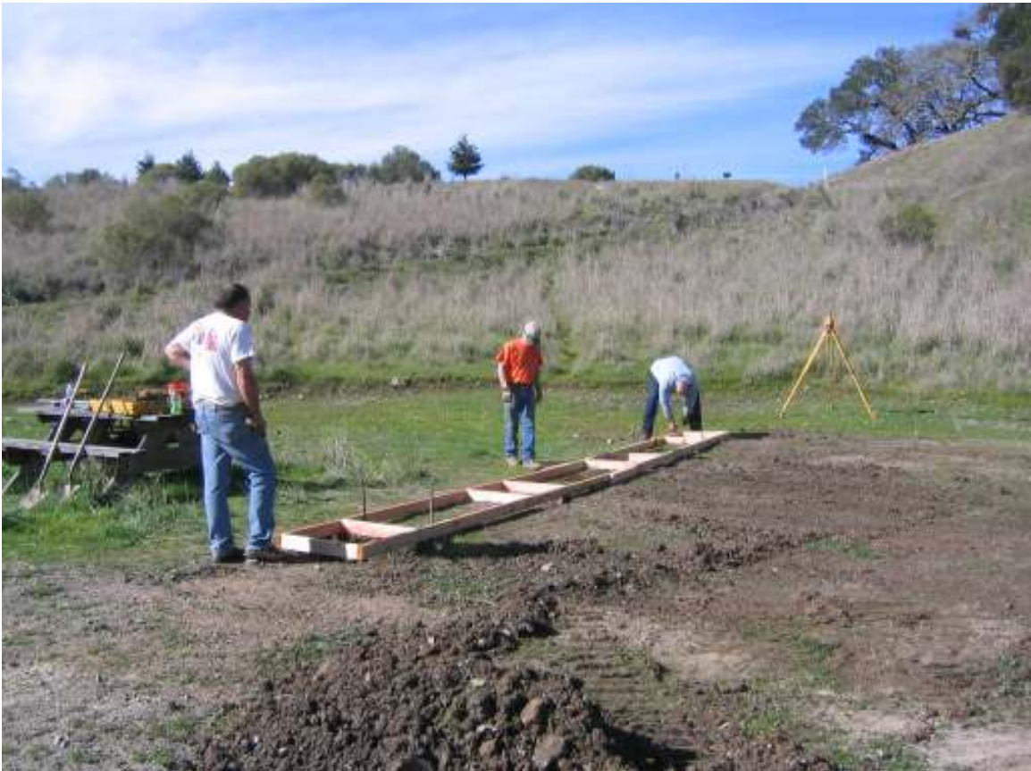
We set up to put in footings for structure
