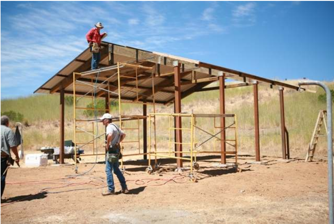
With the trusses up, on goes the roof
